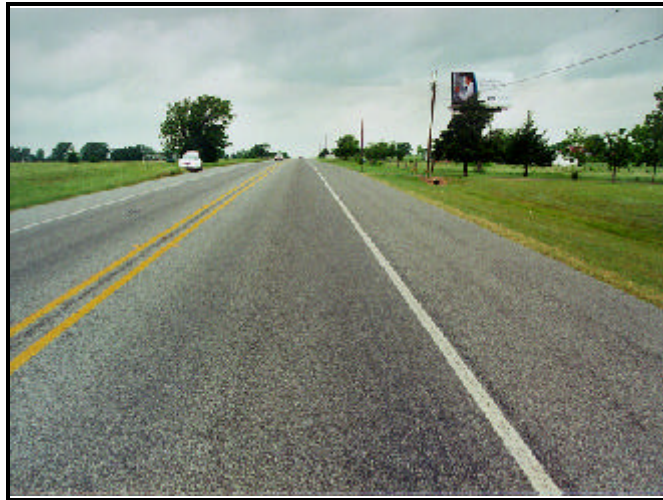
Figure 1. Approach to impact area for case vehicle--facing west.
