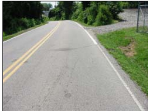
Figure 4. Northbound view of area of impact.
