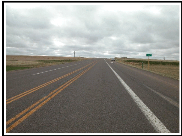
Figure 1. Approach to area of road departure (west)
