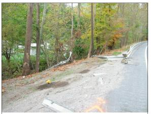
**Figure 14:** Damage to roadway's northern longitudinal barrier caused by overturned Peterbilt tractorsemitrailer; Note: contact damage to trees on northern roadside (case photo #06)
