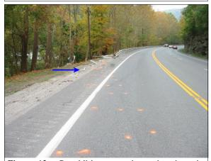
Figure 13: Peterbilt's eastward travel path as it rolled over, landing primarily on the northern shoulder, while continuing to travel forward, impacting and damaging the northern guardrail; Note: arrow shows western-most guardrail support post (case photo #04)
