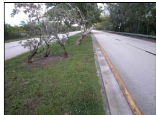
Figure 2. Eastbound approach showing struck tree
