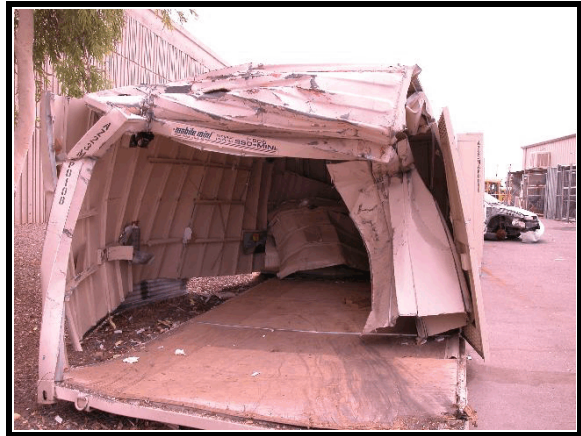
Figure 4. First metal storage structure
