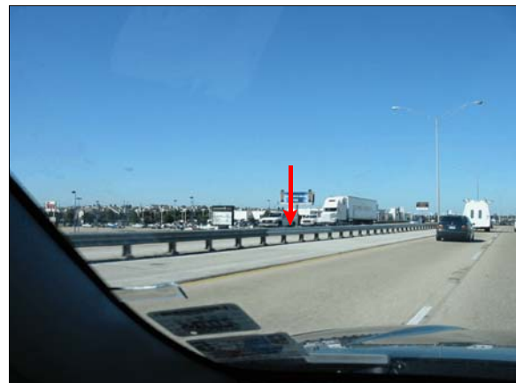
Figure 3: Overview of median guardrail impacted by case vehicle, arrow shows new section of guardrail indicating likely area of impact
