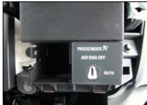
Figure 13. Manual cut-off switch.
