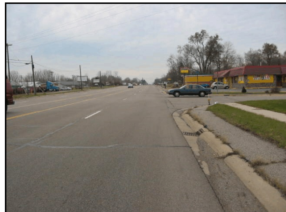
Figure 2: Dodge's westbound approach
