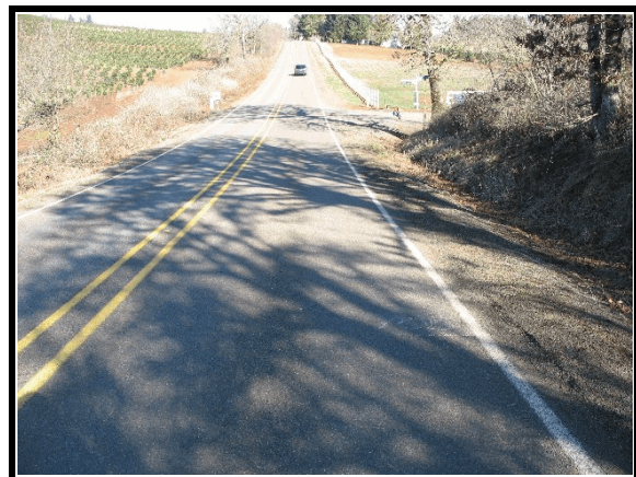
Figure 2. Approach to area of impact
