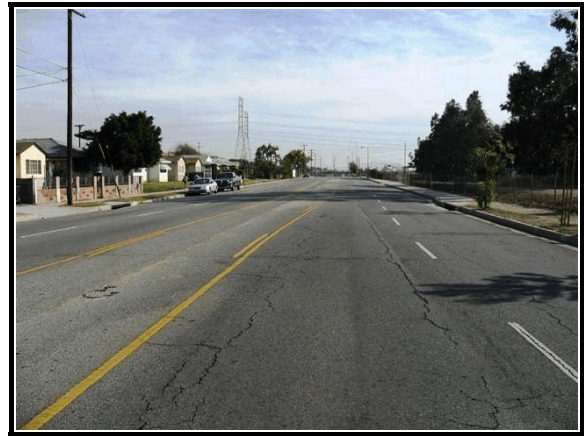
Figure 2. Crash site, southbound approach
