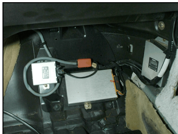
Figure 5: Front right foot well with carpet and panels removed, revealing electrical system components
