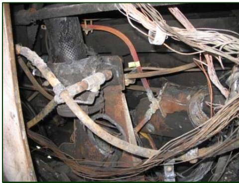
Figure 16. Fuel filter, starter, and starter cables viewed through right side access door.
