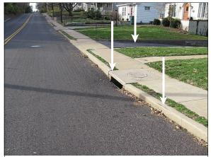
Figure 6: Arrows in foreground show marks on the curb from the impacts by the right front and right rear wheels of the Mazda; arrow in background show final rest position of the Mazda
