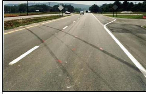
Figure 3. CCW yaw marks across travel lanes.
