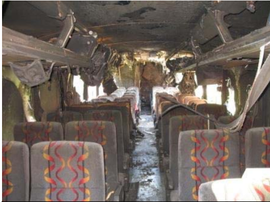
Figure 14. Interior view of the motorcoach looking front to back.
