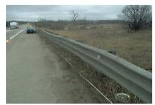
Figure 3. View of the impacted thri-beam guardrail
