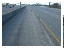
Figure 5. CCW arc of the left side yaw marks.
