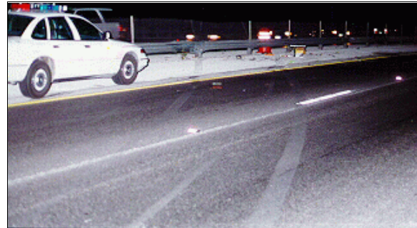
Figure 5: On-scene photo showing case vehicle's travel path into median's guardrail on north roadside during counterclockwise rotation; Note: tire scuffs and damaged guardrail (case photo #05b)
