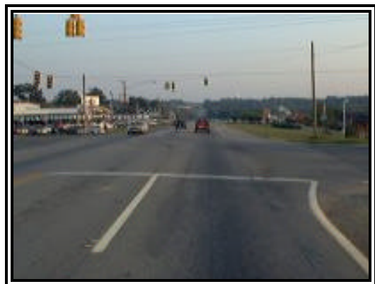
Figure 1: Southward view into the intersection.
