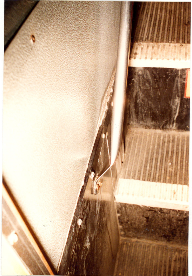
6. Lower handrail attachment point.
