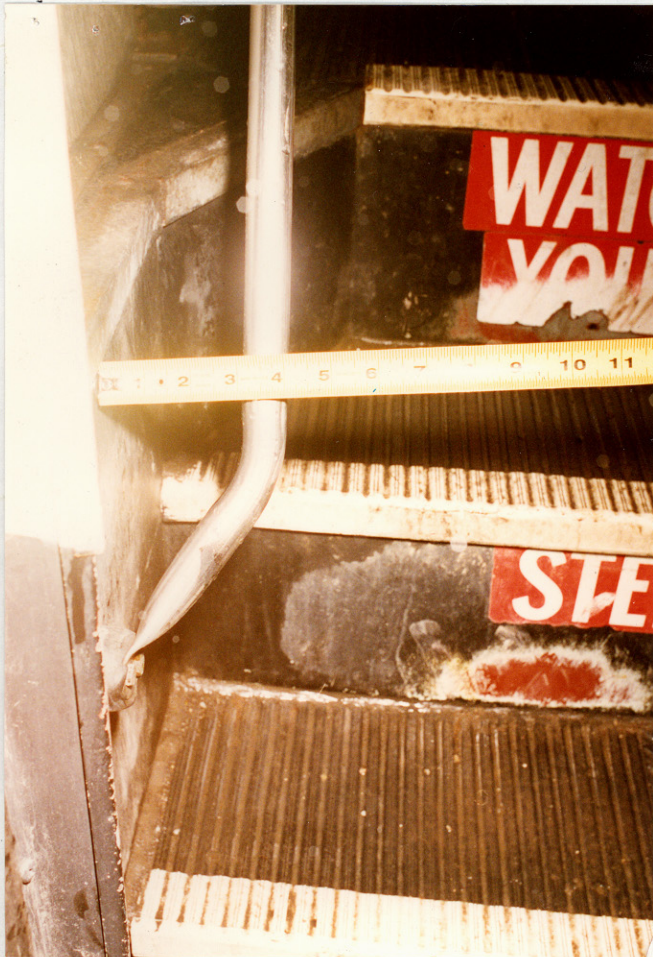
5. & 6. Post-accident retrofitted rubber bushing at the lower attachment of the handrail.
