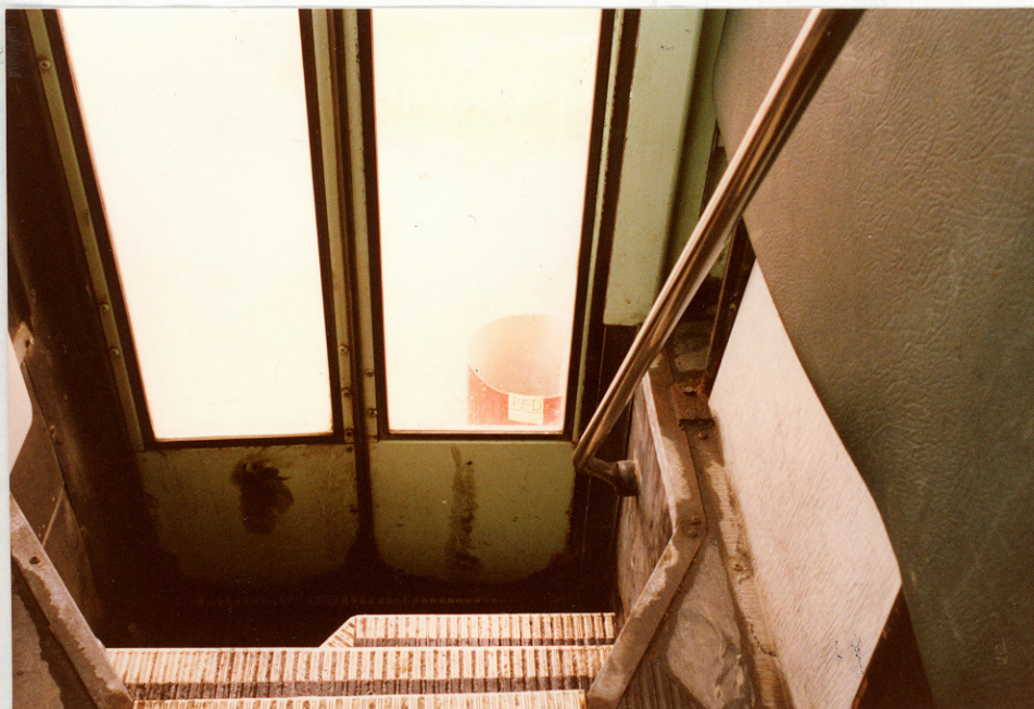
7. Interior view of the post-accident modified handrail.
