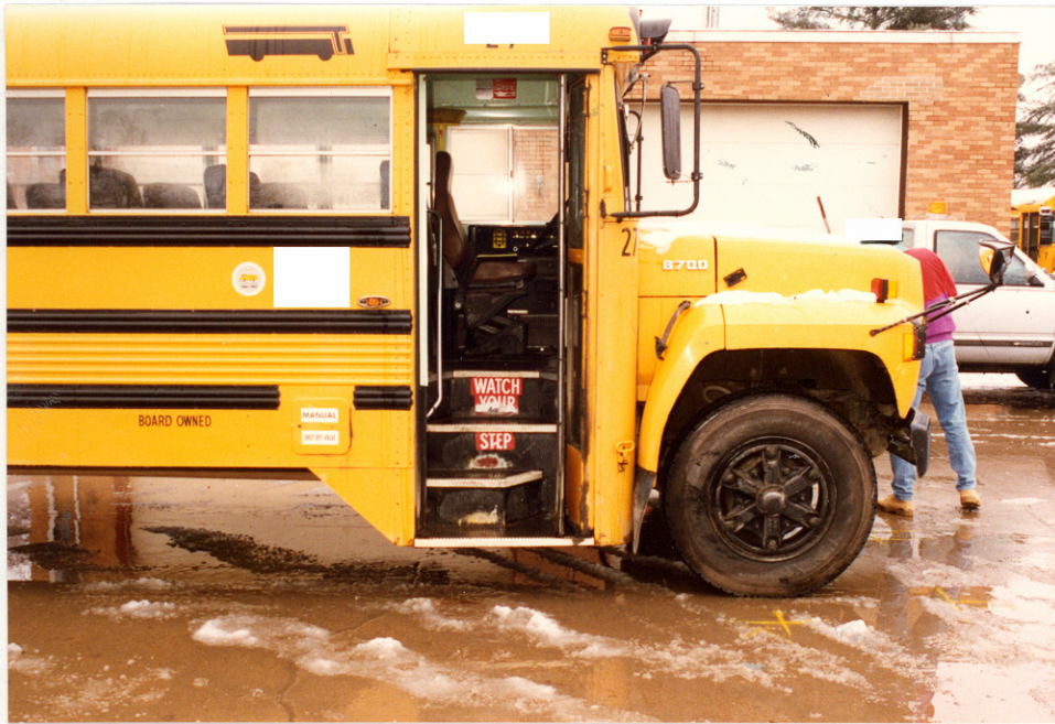
3. Door, stairwell area of the involved bus.
