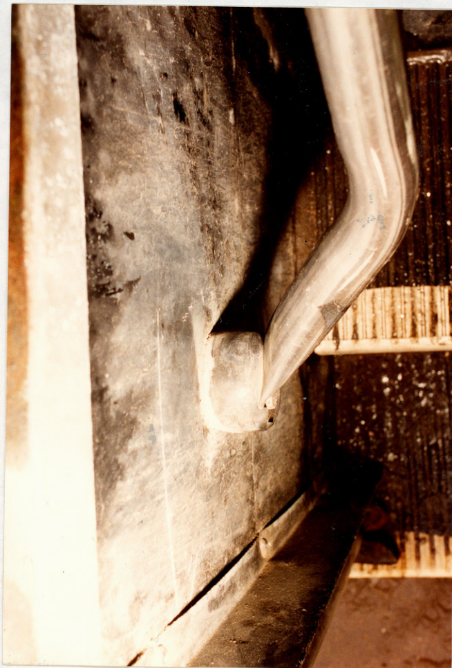
5. & 6. Post-accident retrofitted rubber bushing at the lower attachment of the handrail.
