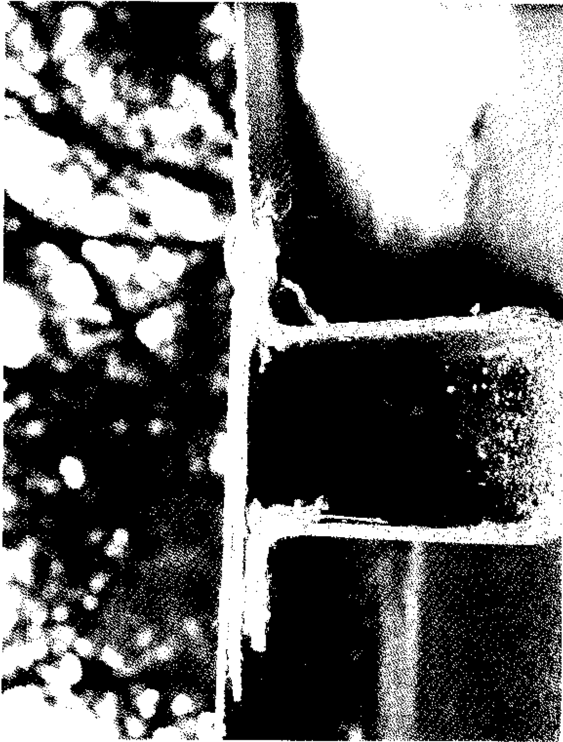
End View of Joint #6
