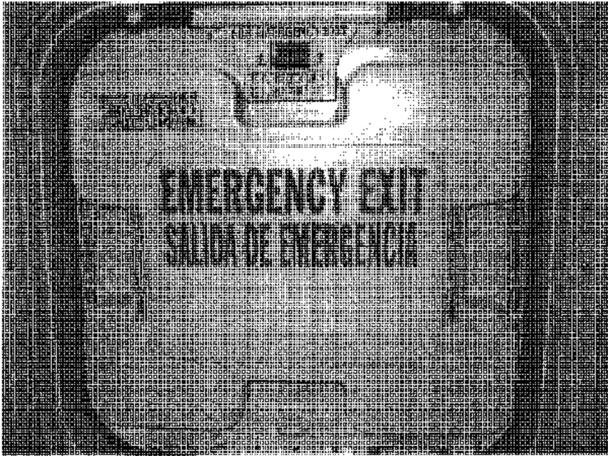
Photo 5 Roof Emergency Exit
