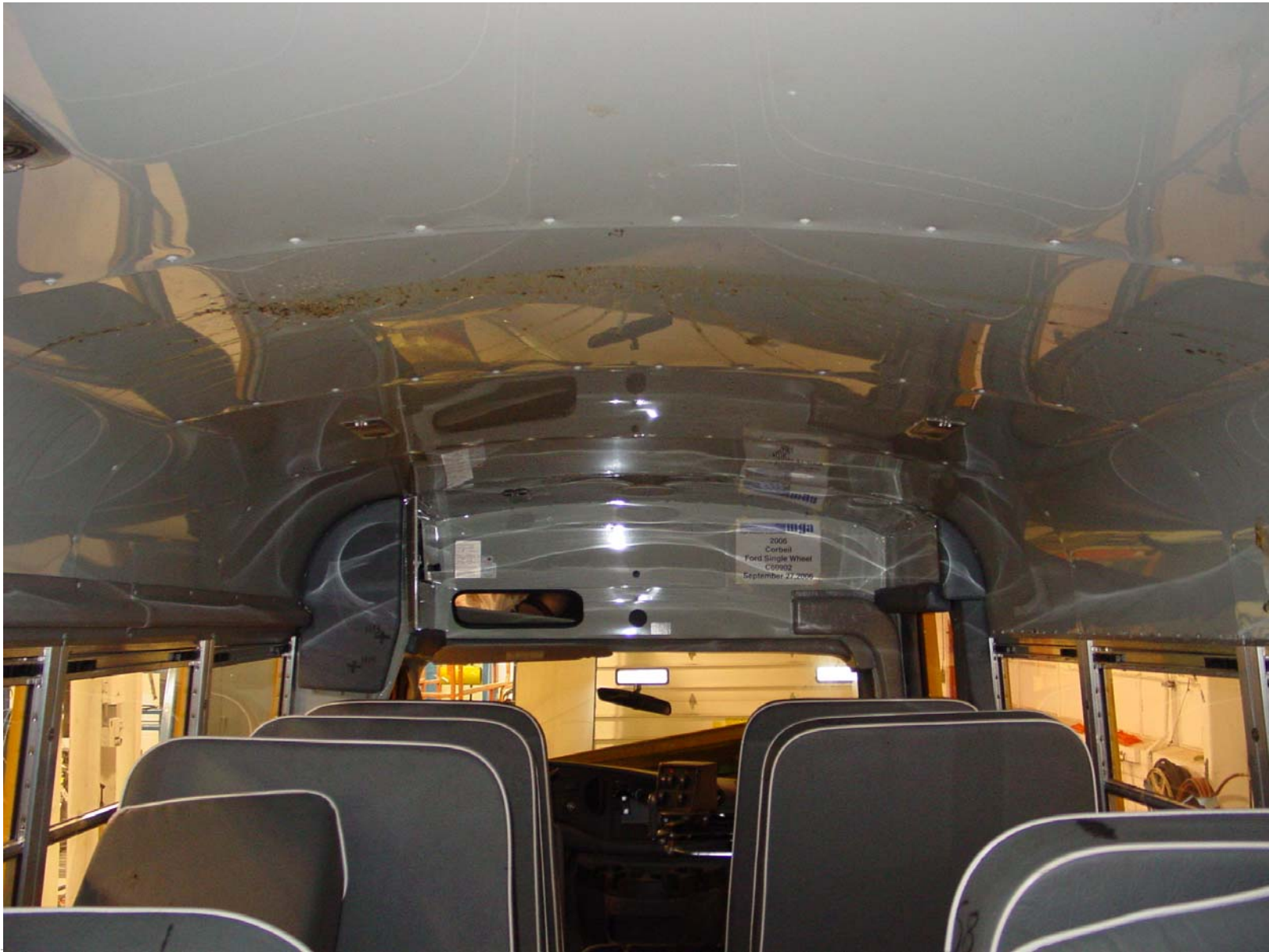
Roof, After Removal of Loading Device, Viewed From Bus Interior
