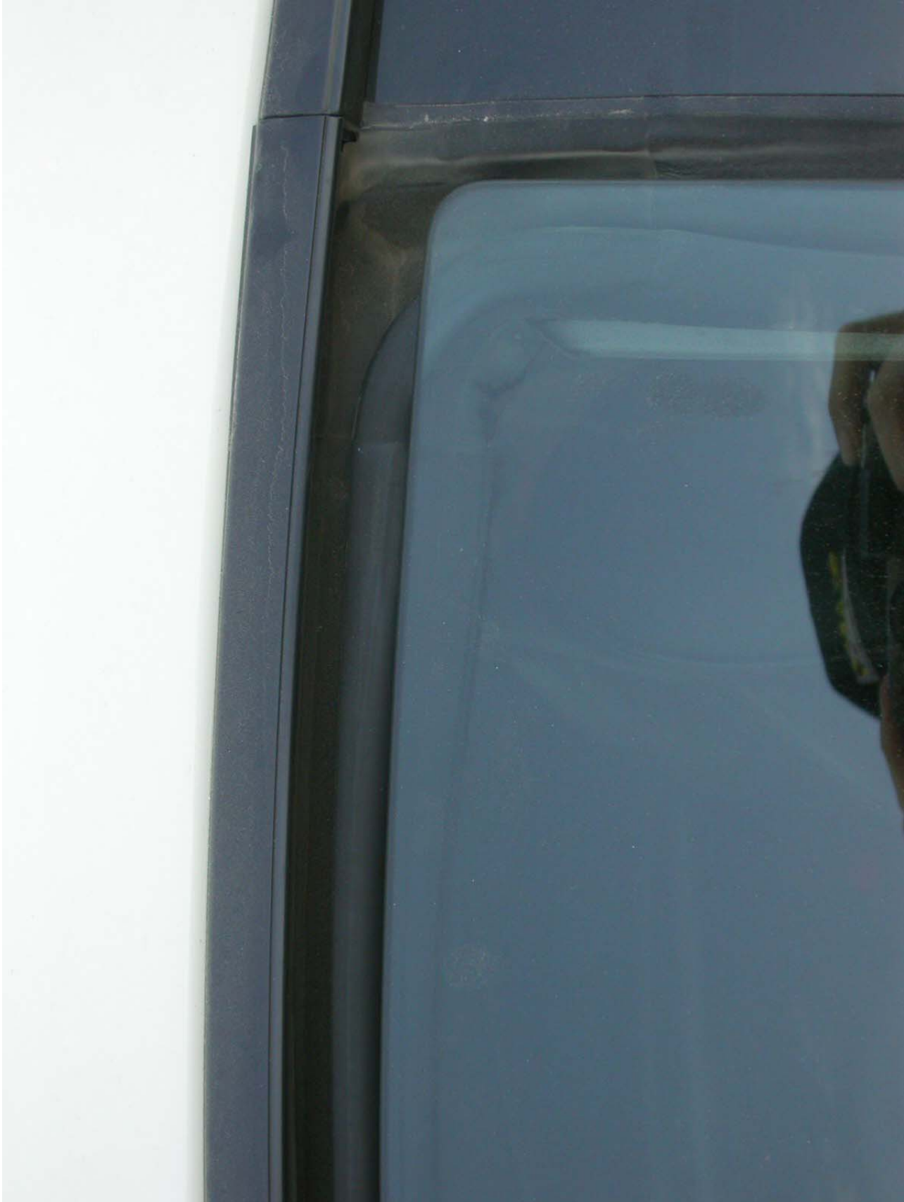
Figure 9: Displacement of Window Indexing on Upper Door Seal
