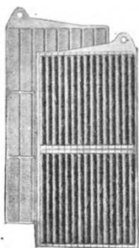
POSITIVE AND NEGATIVE OF EDISON TYPE ACCUMULATOR.
