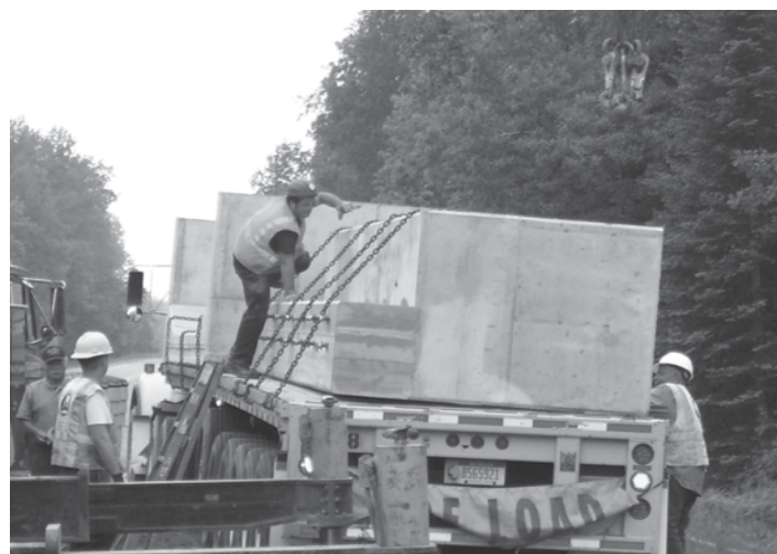
Using precast bridge elements saved time on the rehabilitation of two small bridges on the Michigan route.
