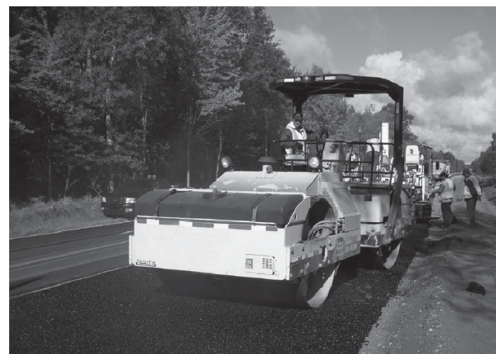
The contractor used an asphalt-stabilized crack relief layer to help meet the five-year pavement warranty requirement.
