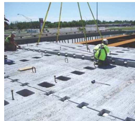
Innovations such as full-depth precast deck panels helped the Iowa DOT save time and money on an interchange project.
