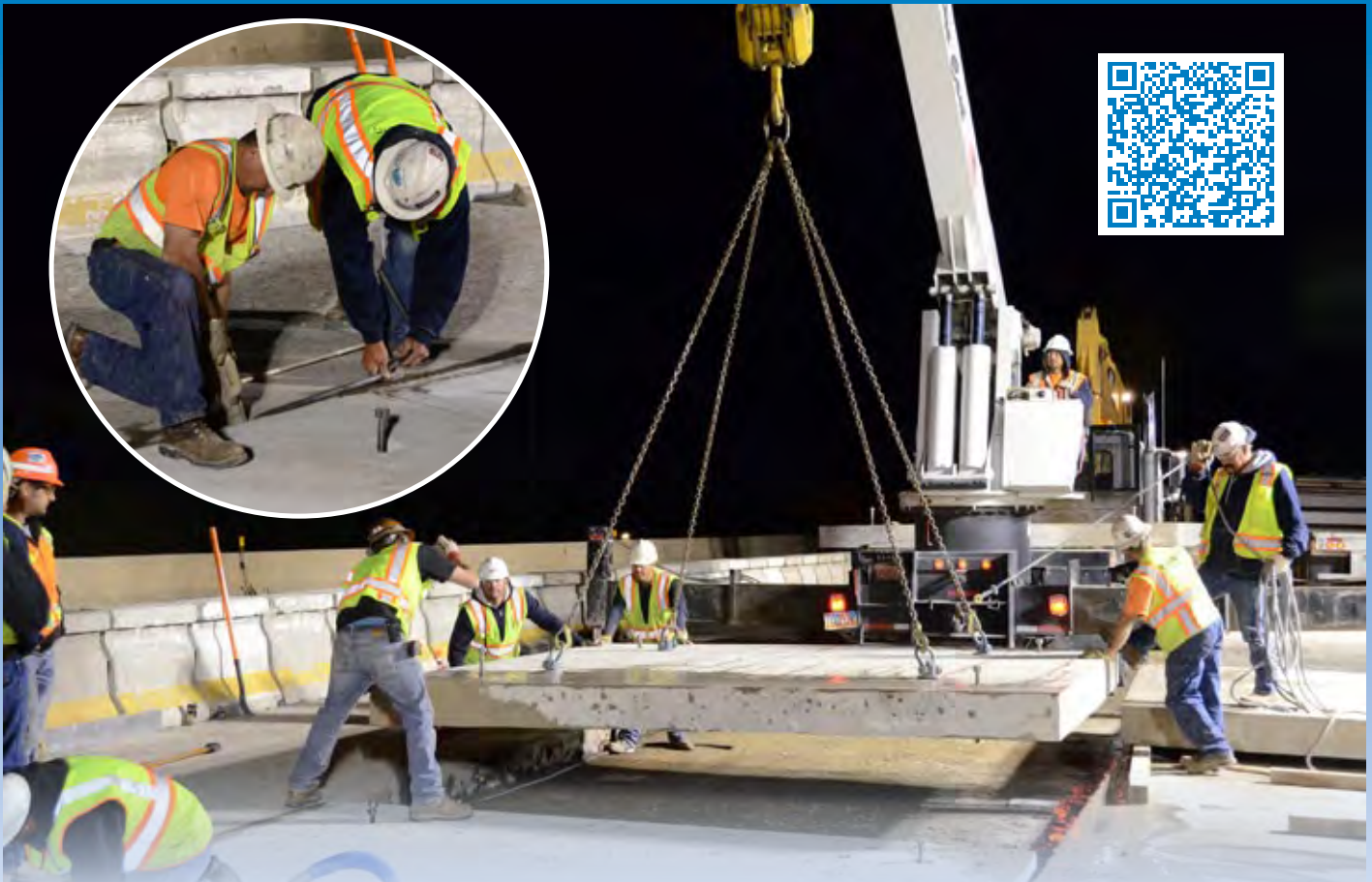
The Utah Department of Transportation demonstrated rapid repair of concrete pavement with precast panels at a Highways for LIFE showcase in Salt Lake City. More than 200 transportation professionals from across the United States took advantage of the opportunity to learn about the design, construction and installation of a new type of precast panels on a section of Interstate 215. The panels speed up the repair process, minimize traffic disruption and boost durability. For more on the showcase, visit www.udot.utah.gov/main/f?p=100:pg:0:::1:T,V:3477 or scan the QR code with your mobile device.
