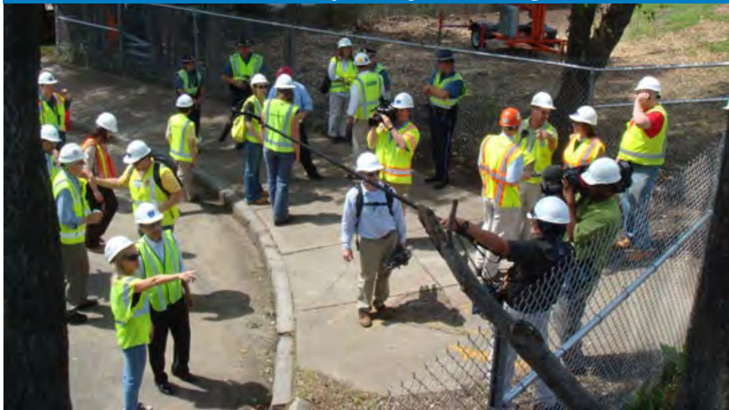
Transportation professionals from around the country came to Medford to observe the weekend installation of a new bridge on I-93 south over Salem Street.
