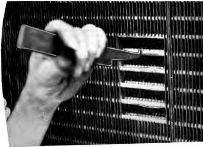
Fig. 90 Closing the Seams on Front of Tubes
