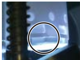
Inspect for cracks in case windows.
