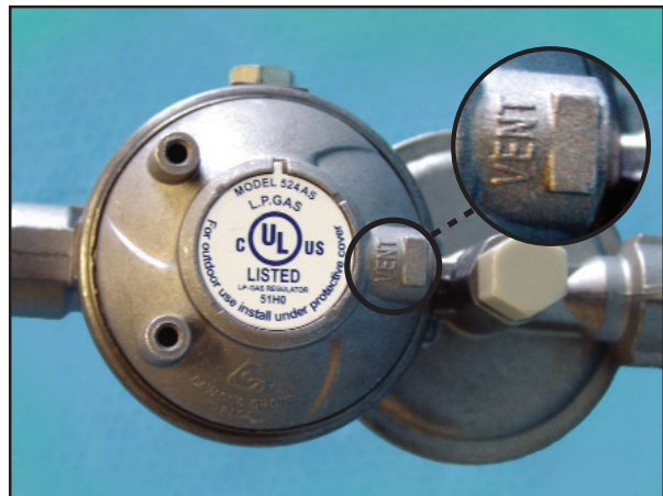
Figure 2 If the regulator's vents face horizontally in the installed position, the regulator is incorrect and must be replaced.
