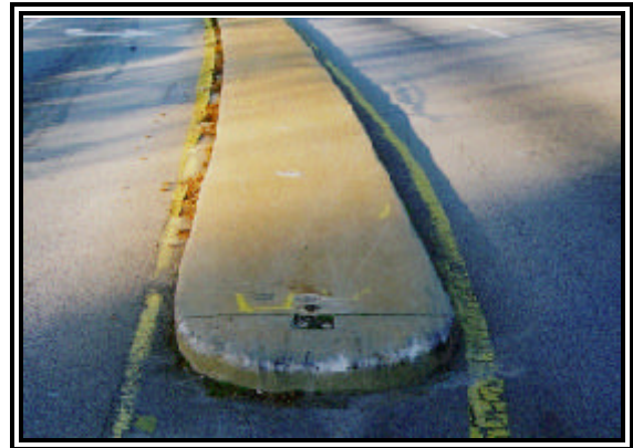
Figure 2: View of the raised median, west of the intersection.
