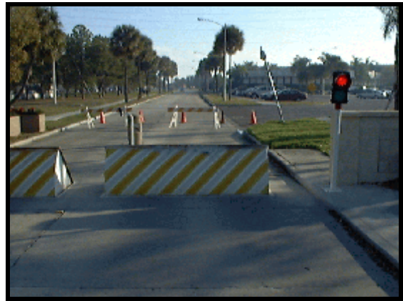
Figure 10: Trajectory view of the security barrier.
