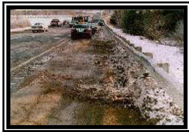
Figure 2. 1994 Geo Prizm impact to W-beam guardrail.
