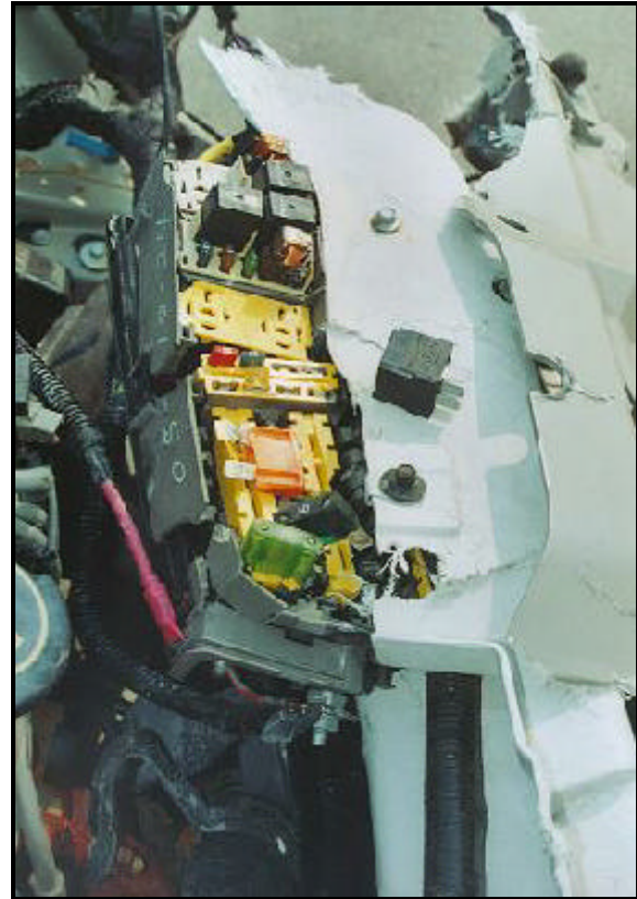
Figure 7. Damaged fuse block
