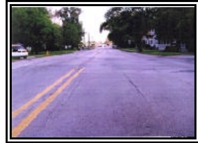
Figure 6. Point of impact showing pre-impact skid marks from the Galant
