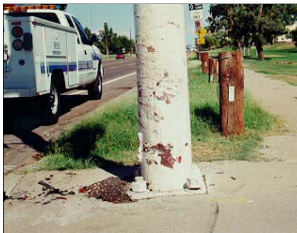
Figure 6: Close-up police photo, taken next day, looking east at metal pole struck by case vehicle (case photo #10)
