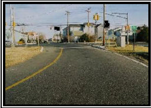
Figure 1. Eastbound approach for the 2000 Infinity I30.
