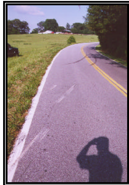
Figure 3: Look back view.
