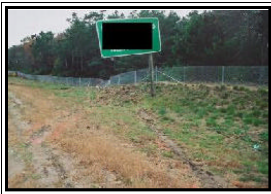
Figure 2. Struck signposts and chain link fence.
