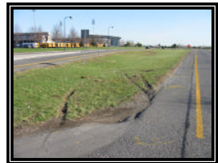
Figure 3. Area of final rest showing gouge marks from the Civic
