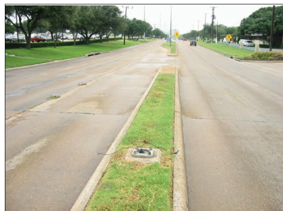
Figure 3: Base of light pole, located in median, that was sheared by contact with case vehicle's left front wheel assembly (case photo #09a)
