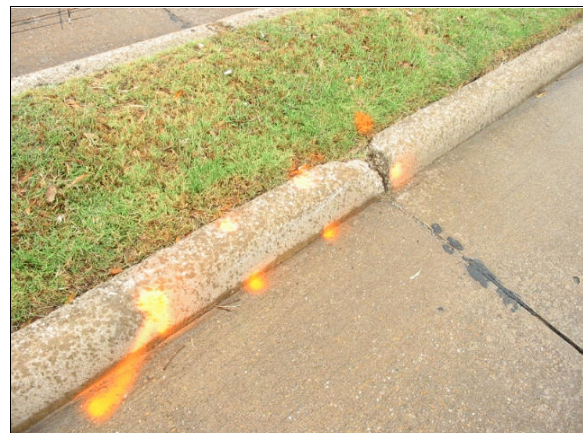
Figure 2: Northeastward close-up view of impact to median curb from case vehicle's left front wheel (case photo #07)
