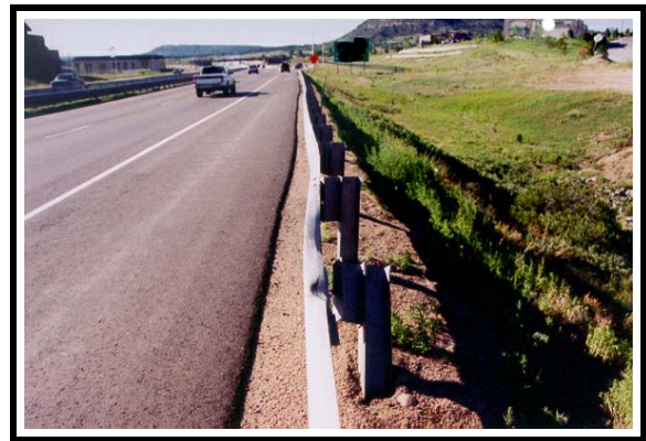
Figure 3. Left side of case vehicle impact top-back side of guardrail and rollover embankment.
