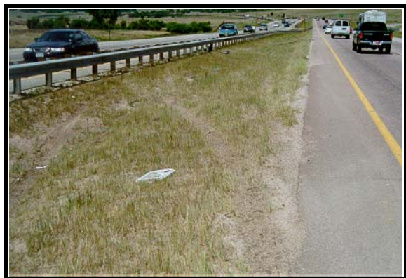
Figure 2. Vehicle path into guardrail (first event)
