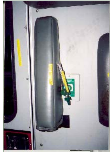
Figure 16. Displaced oxygen valve.
