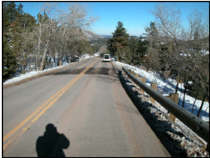
Figure 1. Approach to area of impact (North)
