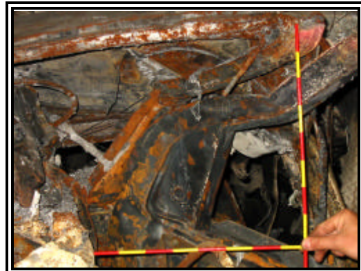
Figure 16. Frontal view of the left A-pillar - Incremented sticks show the lateral displacement of the lower aspect
