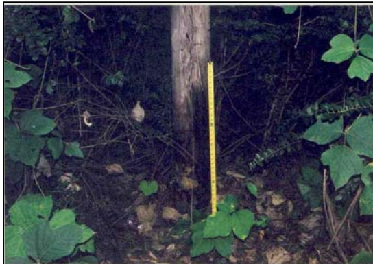
Figure 3 - Impacted utility pole (Event 1).
