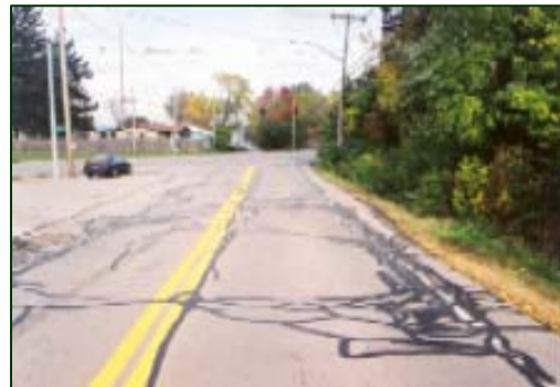
Figure 2. Overall view of the crash site from a northerly direction.
